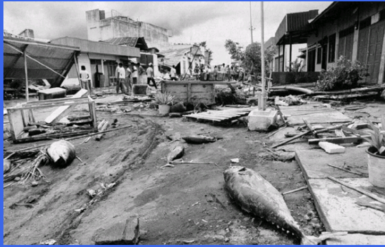
Tsunami damage in Indonesia (1992)
