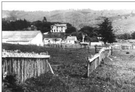
A fence built across the San Andreas fault near Bolinas, California, is offset by nearly 3 m after the great San Francisco earthquake
