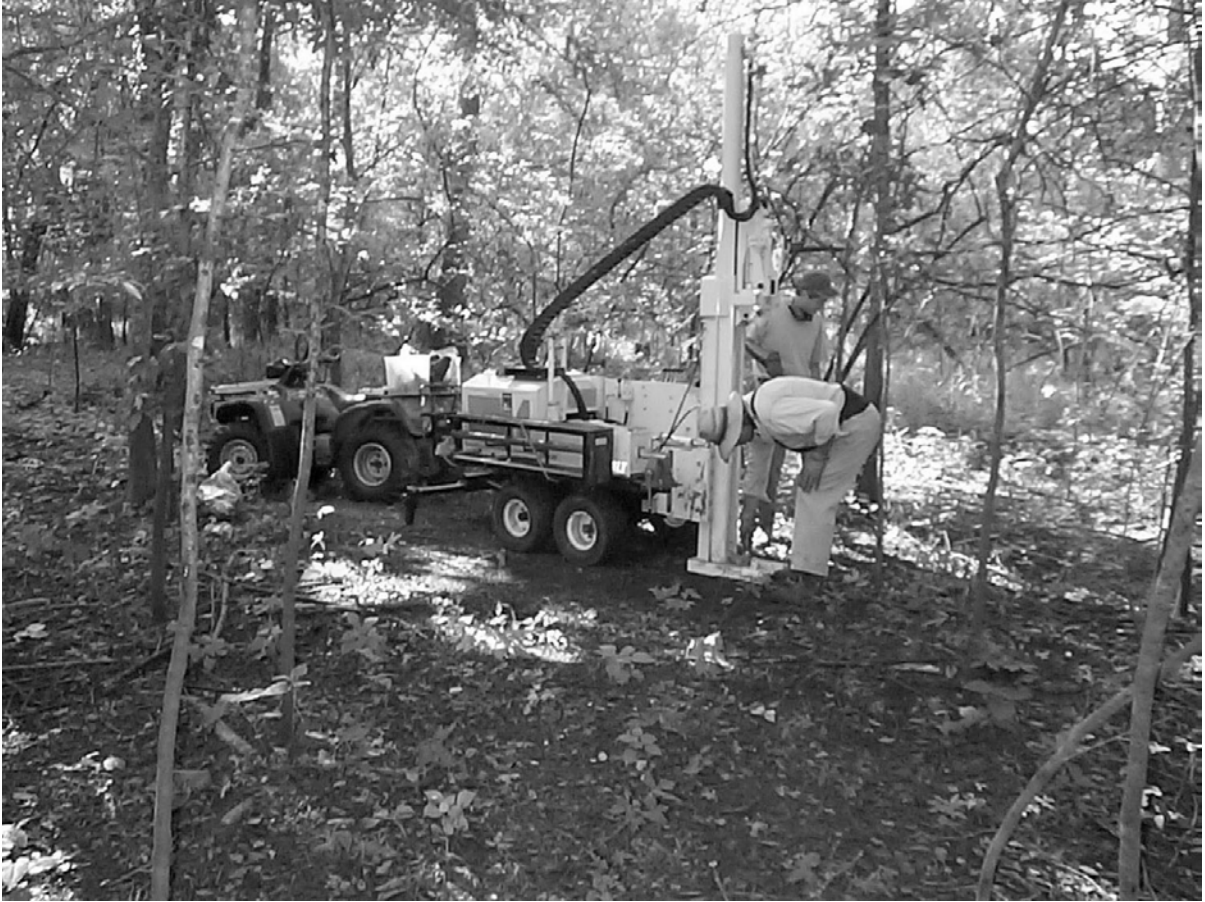
Figure 5-1. Coring in progress at Location C-1. Facing South. Date:9/5/03.
